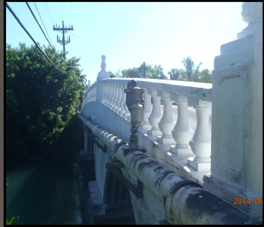
Overhead Electric and Bridge Mounted Utilities
