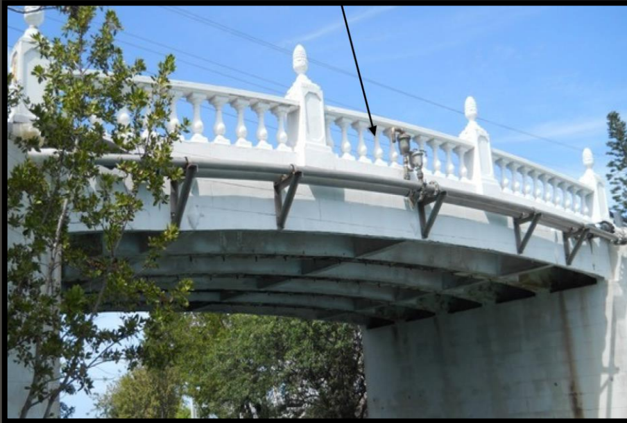
Bimini Drive Bridge
