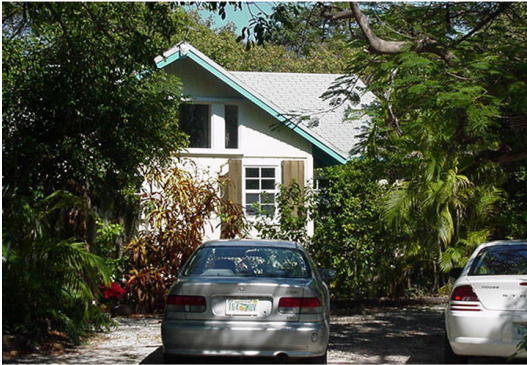
178 Beach Road - Built 1941 - RE 90270.000202 - MO03643 - 1/05
