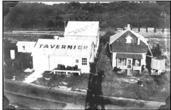
Figure 10 Railroad-Oriented Buildings (demolished)
