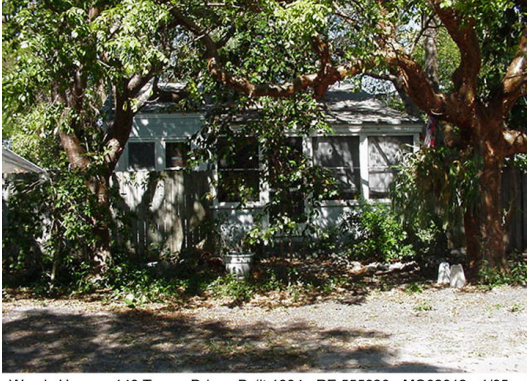
Woods House - 140 Tavern Drive - Built 1934 - RE 555820 - MO02012 - 1/05
