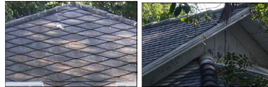
Figure 20 Composite Tile and Clay Roofing
