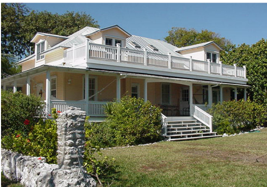
200 Beach Street - Built 1935 - RE 557120 - MO01985 (?) - 1/05
