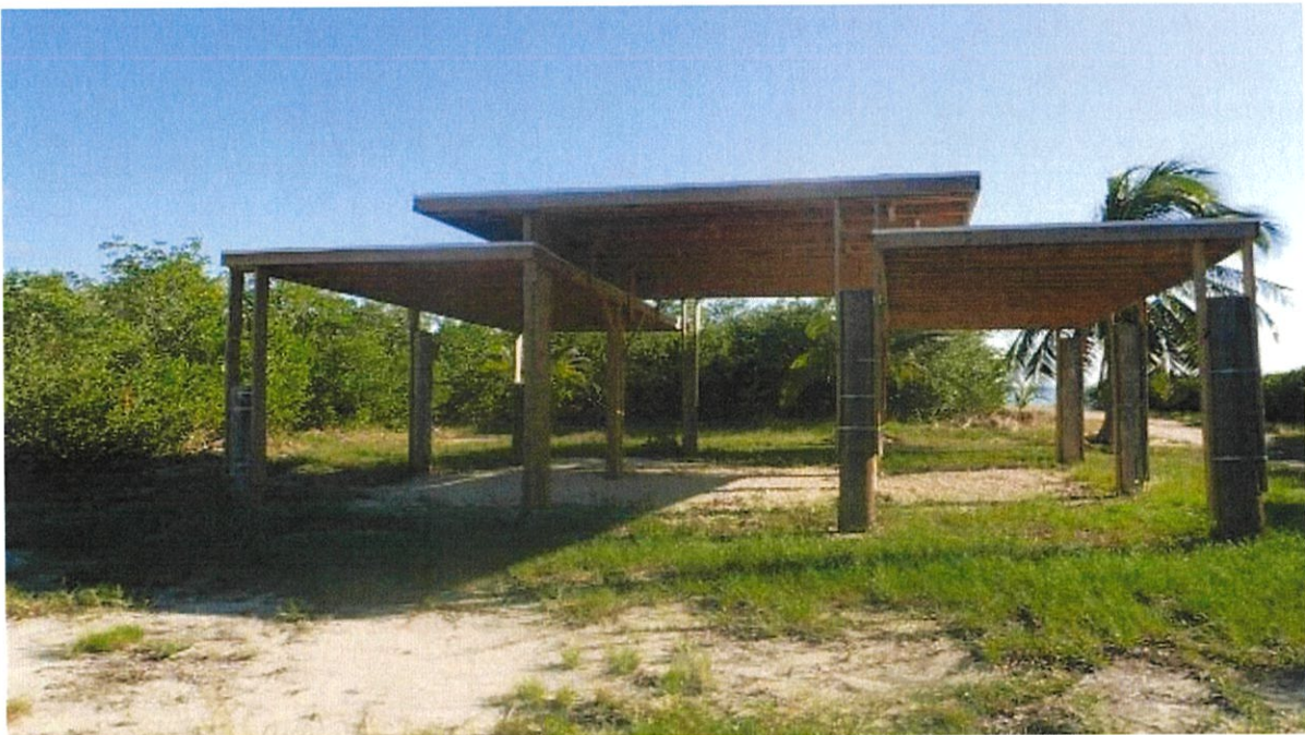
Site conditions, Lot 16, showing the accessory structure with mangrove in the background.
